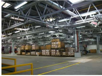
BMW AG, Logistikhalle
