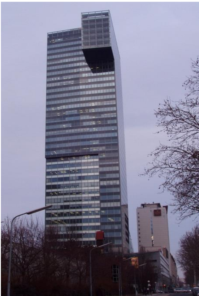
Innenausbau IZD-Tower Wien
